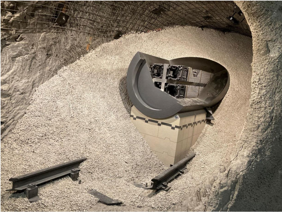
Image 6: Scale model for the storage of spent fuel elements. Copyright: Henriette Herzog/AGES
